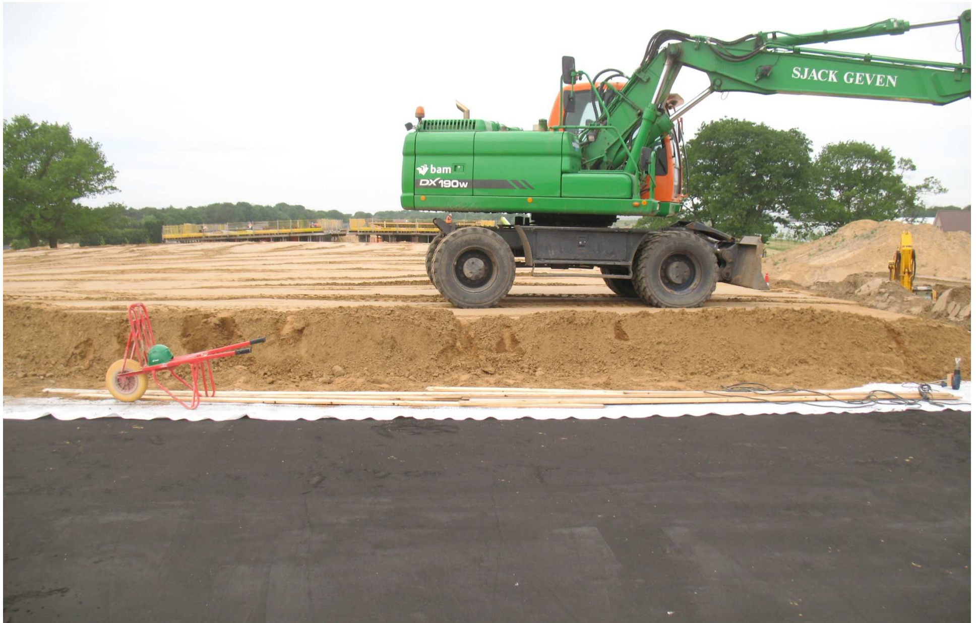
Highway Greenpoort Lane construction - waste slag capping (100.000 m 2 ), Venlo, the Netherlands 2011
