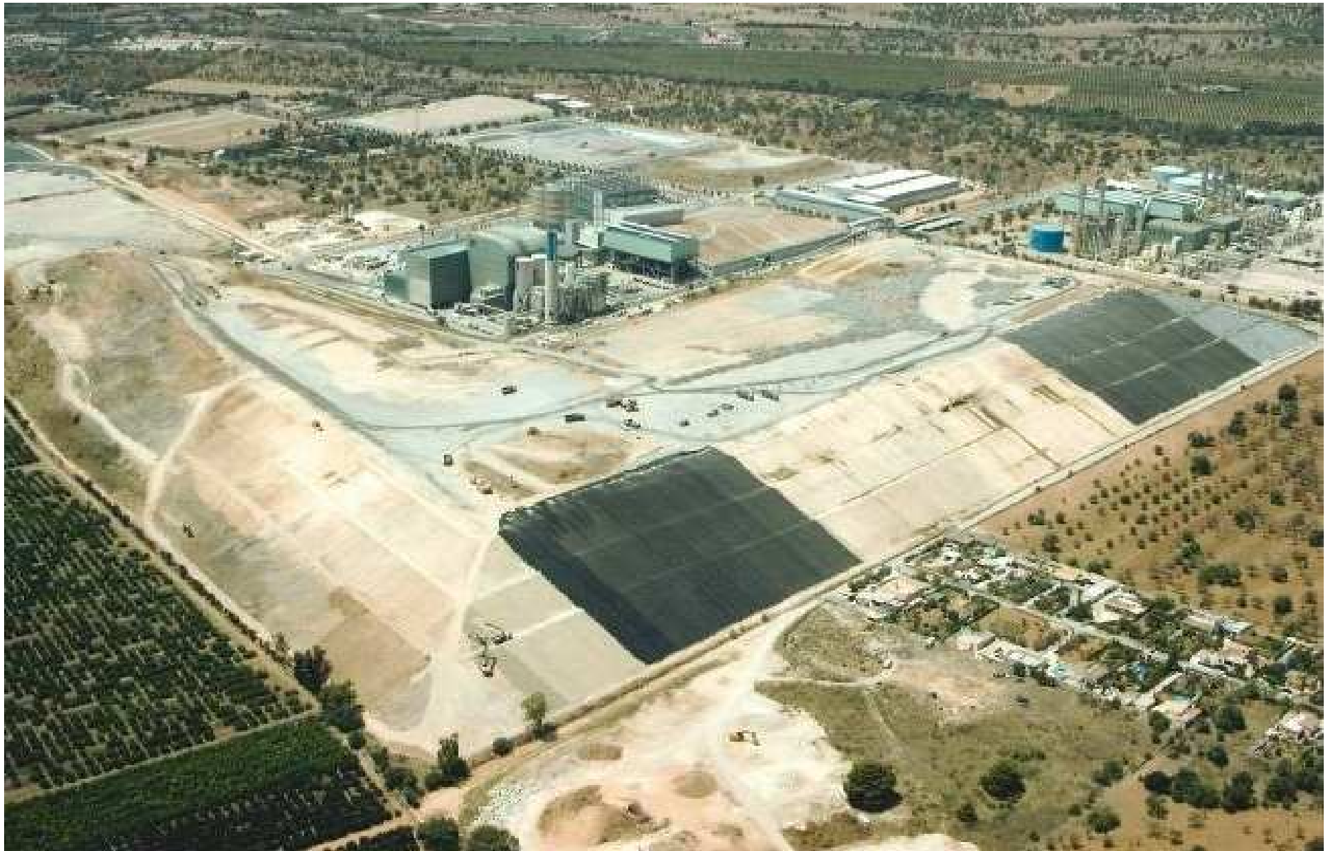
Landfill capping (310.000 m 2 ) Son Reus, Mallorca, Spain 2010
