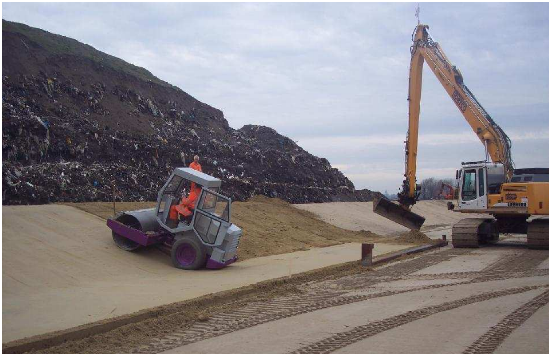
Deponije - fundament deponije opasnog otpada (15.000 m 2 ) Heiloo, the Netherlands 2008
