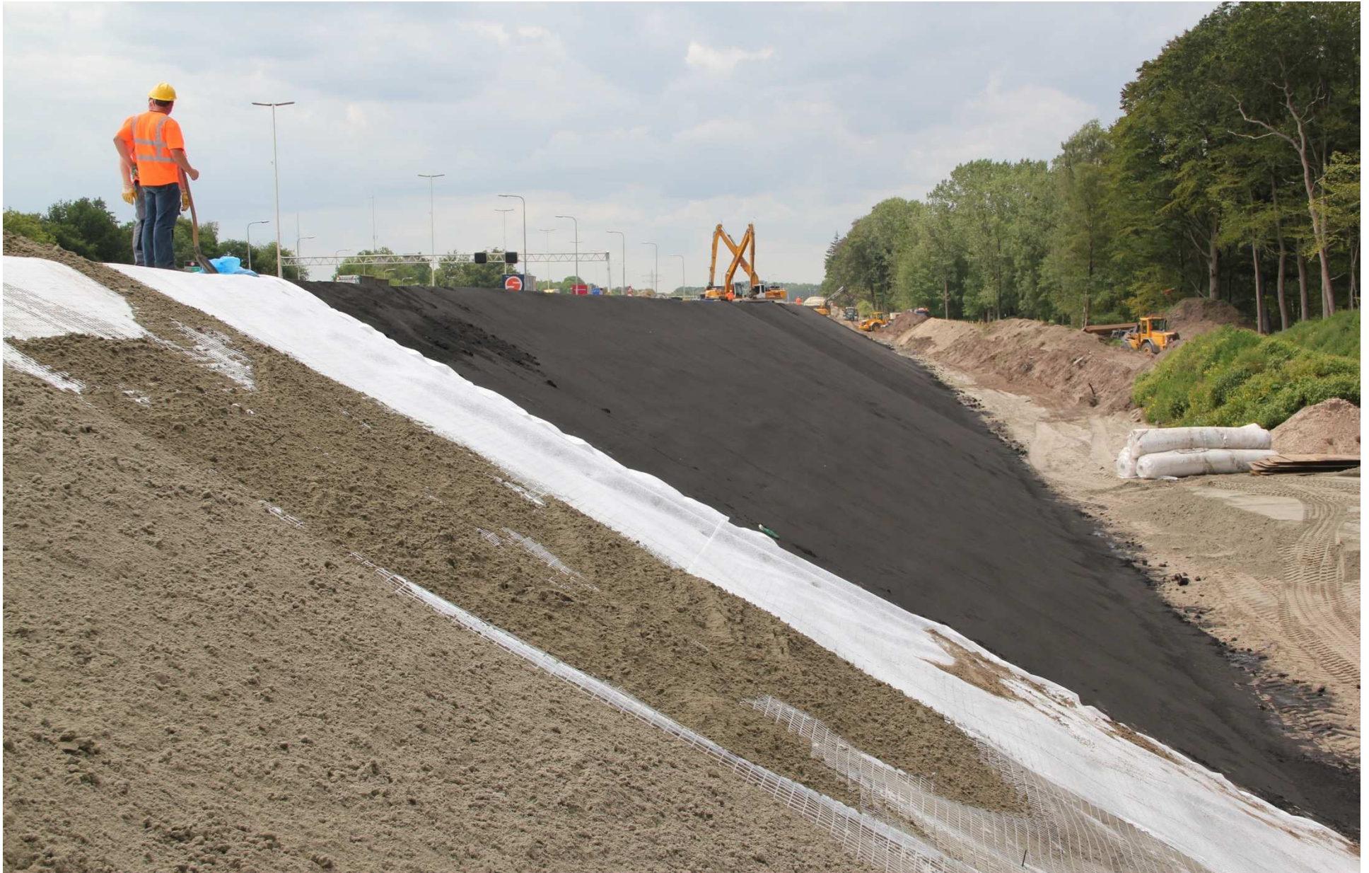
Highway Veenendaal construction - waste slag capping (100.000 m 2 ) Veenendaal, the Netherlands 2011
