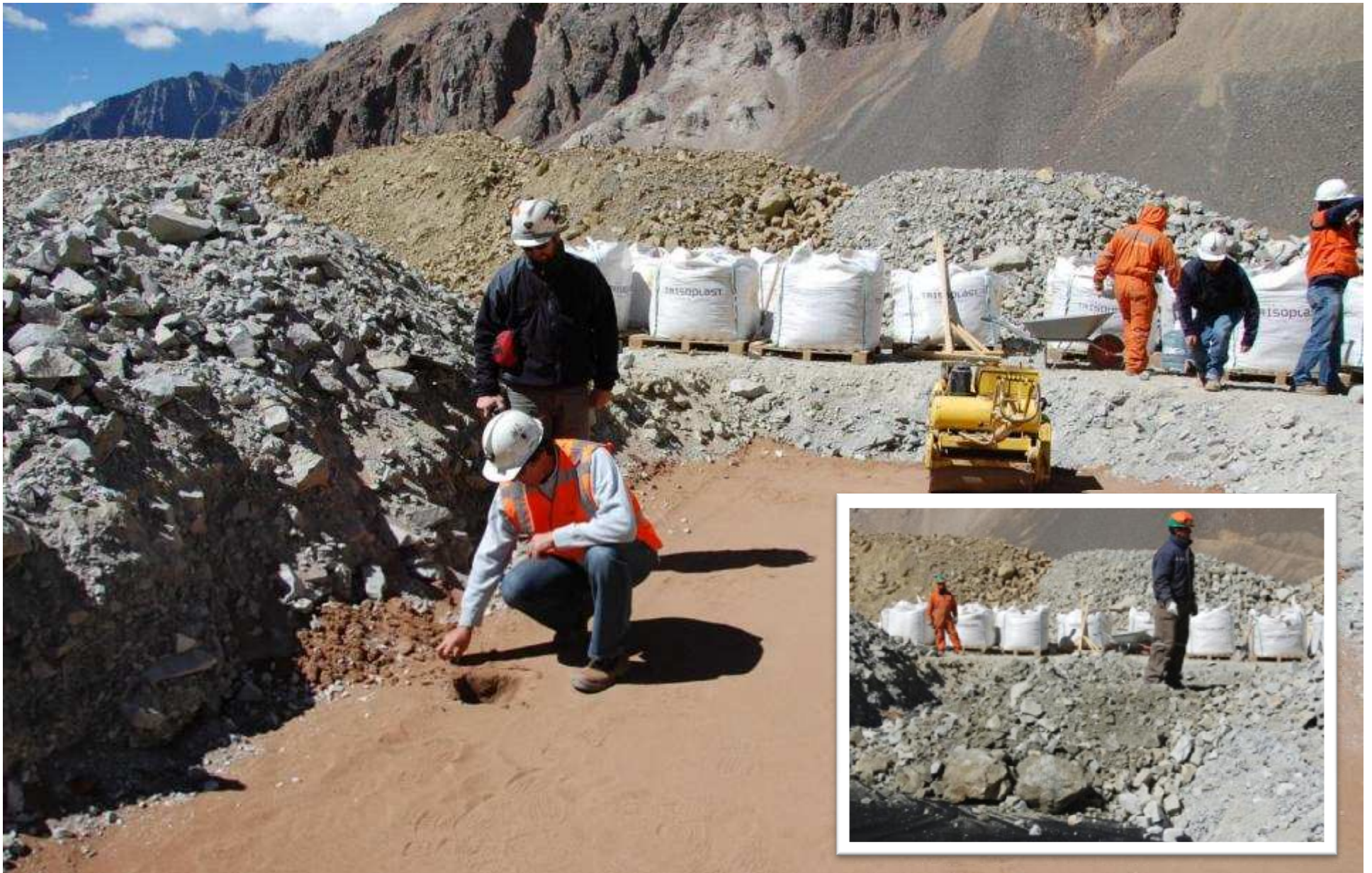
Liner for meltwater flow area at copper mining site (1.000 m 2 ) Los Andes, Chile, 2010
